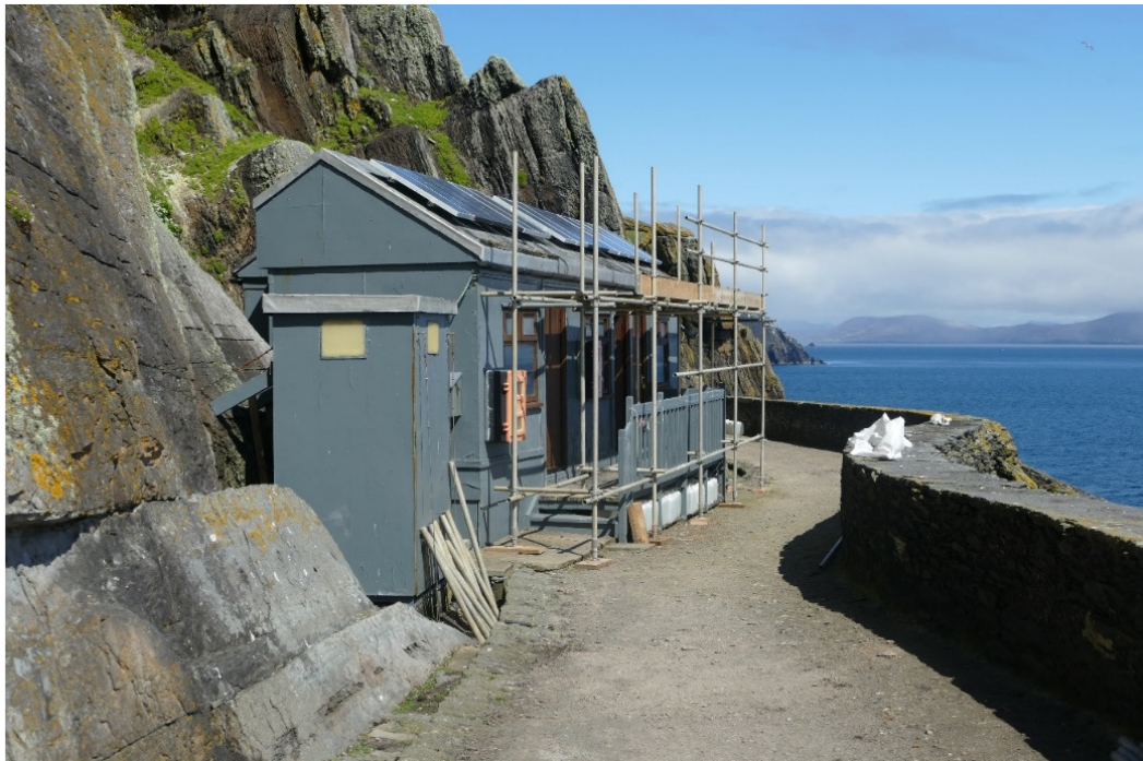
Figure 19 - New solar panels installed to guides huts on site
