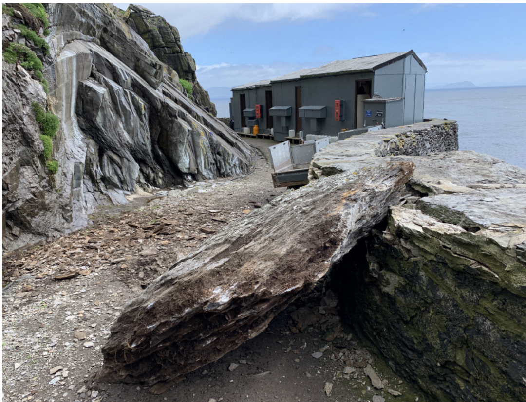
Figure 27 - Rock Fall on 27 th July 2020
