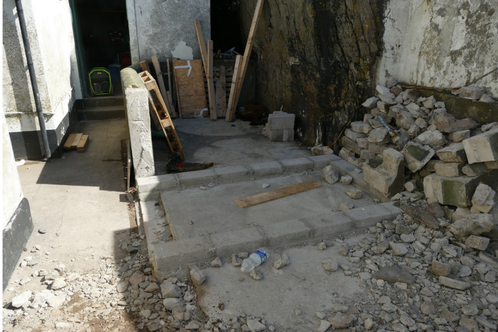
Figure 13 - Foundation for the proposed composting toilet installed at the Lower Lighthouse compound
