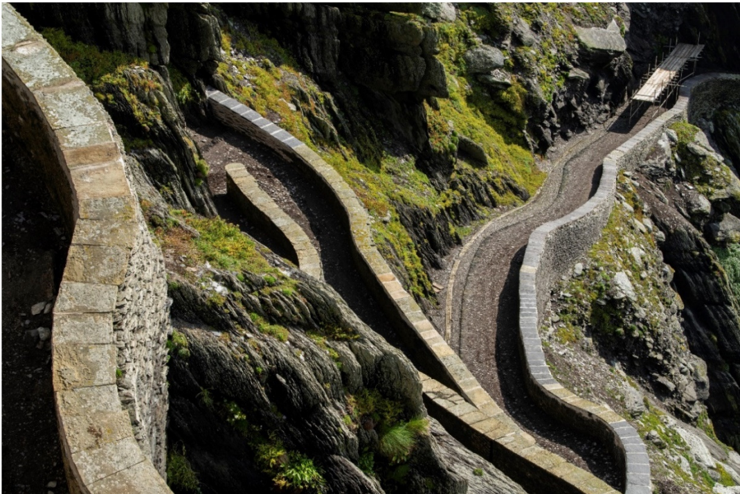
Figure 8 - View of the Upper Lighthouse Road from the Upper Lighthouse gate © Photographic Archive, National Monuments Service, Government of Ireland
