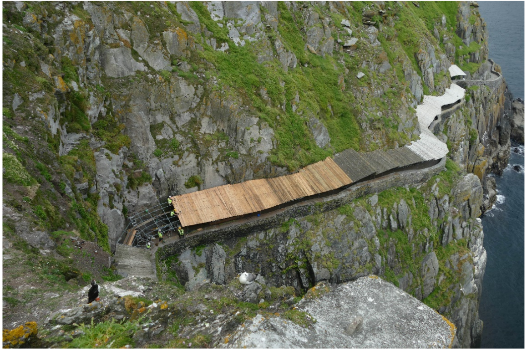
Figure 34 - Timber repairs in progress to Crash Deck at Cross Cove
