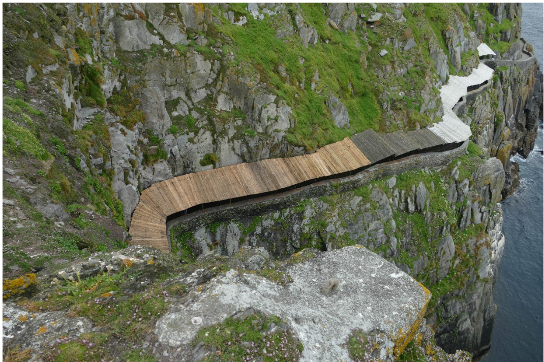
Figure 35 - New Timber decking installed on Crash Decks at Cross Cove
