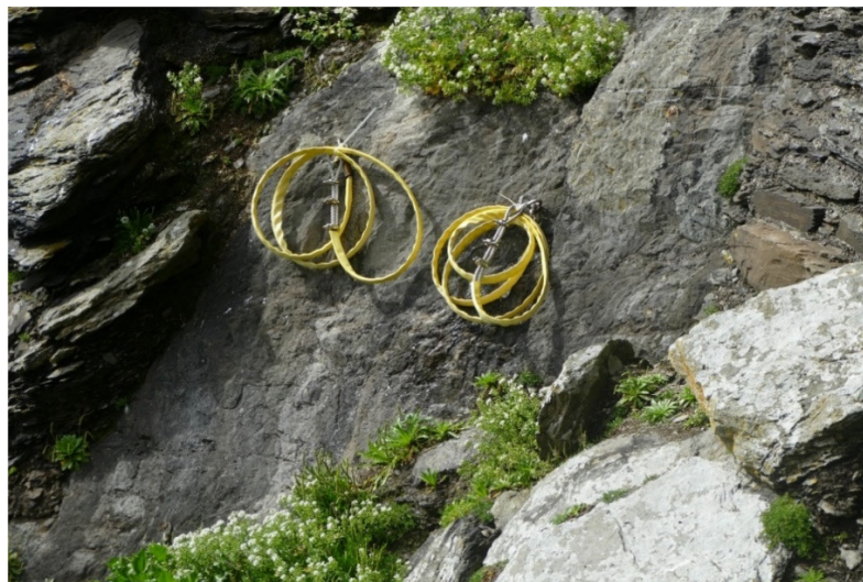
Figure 29 – View of the stainless steel stays coiled up and attached to the rock face below the sea walls
