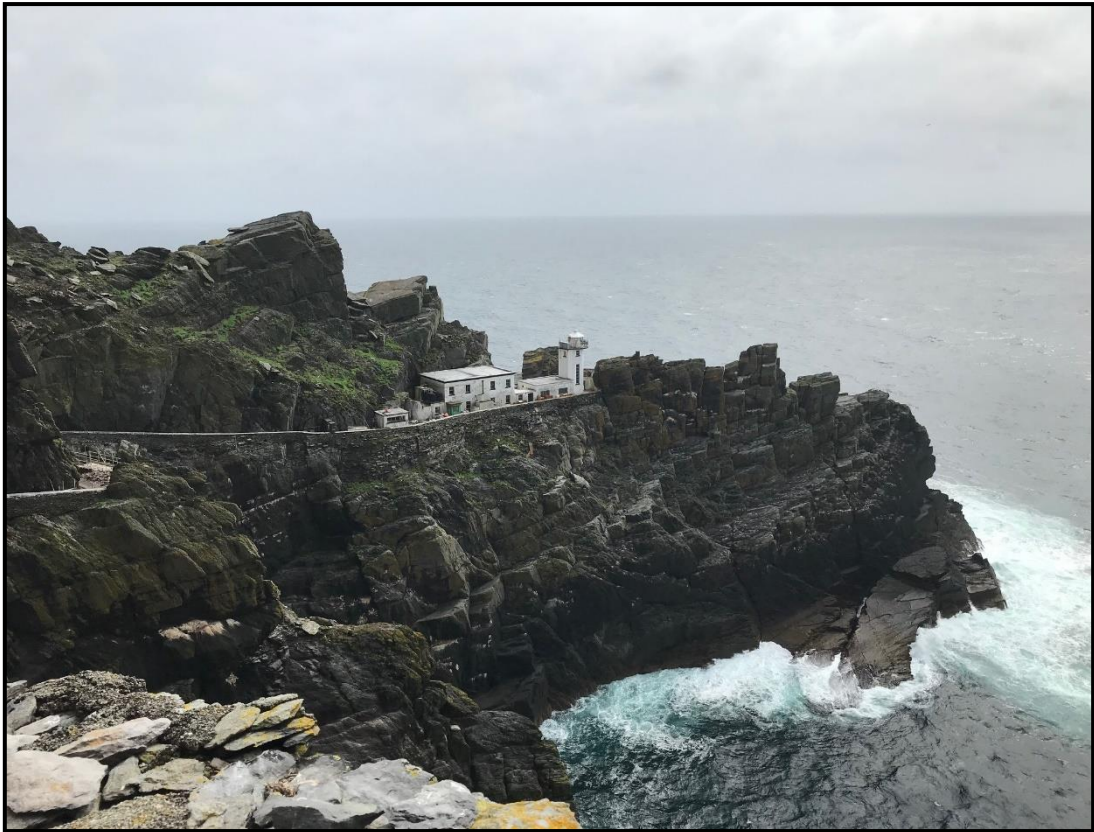
Figure 3 The Lower Lighthouse at Seal Cove
