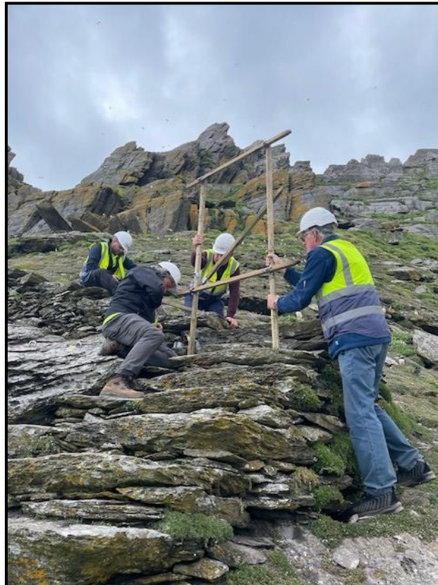
Figure 5 OPW personnel using a timber template to assess potential for handrail at location on south steps.
