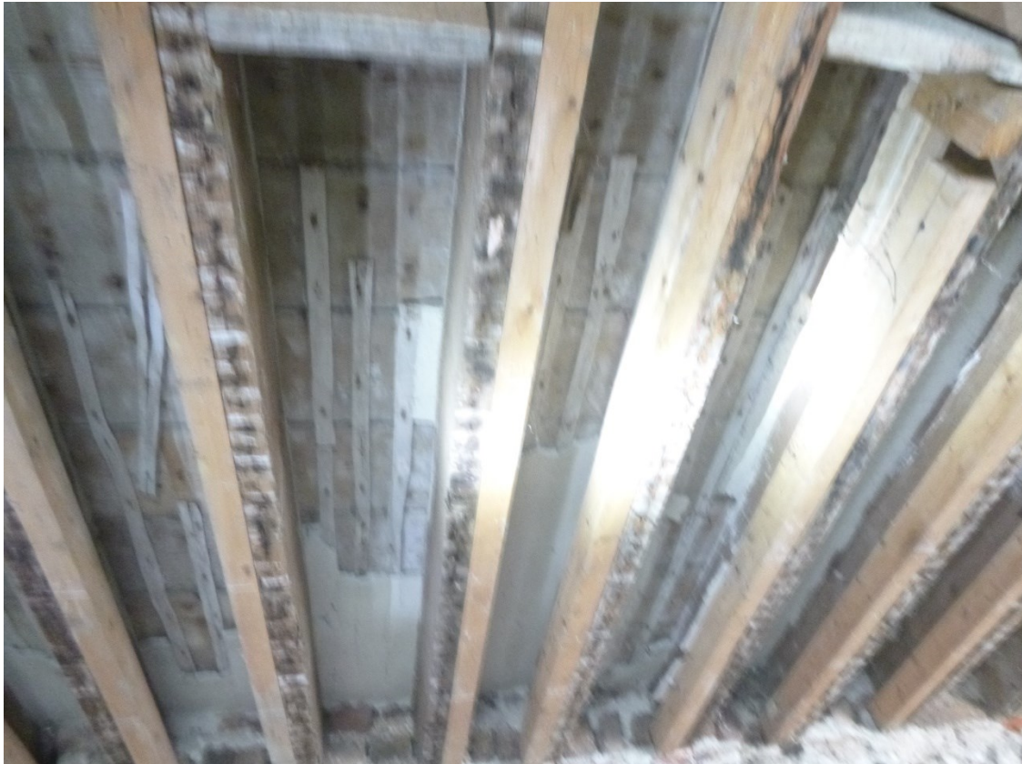
Photo 12: View of underside of first floor timber joists
