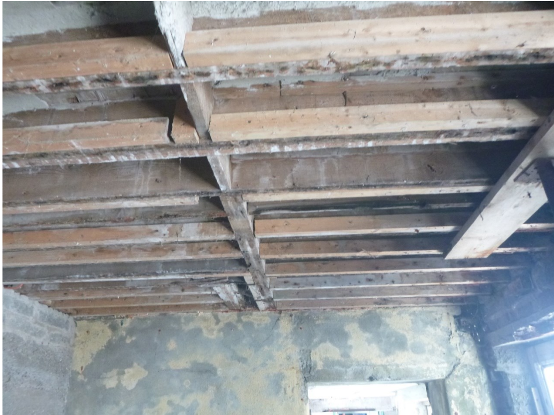
Photo 11: View of underside of first floor timber joists
