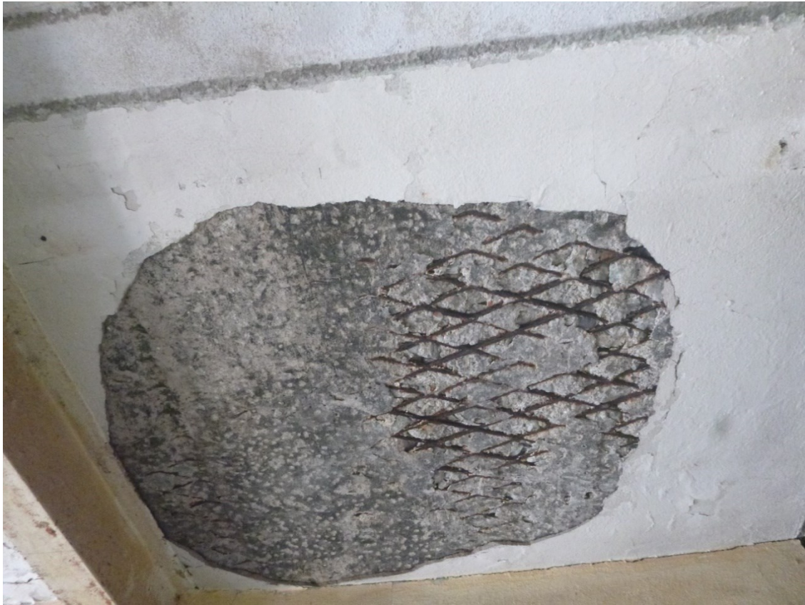
Photo 15: View of expanded metal in first floor roof slab
