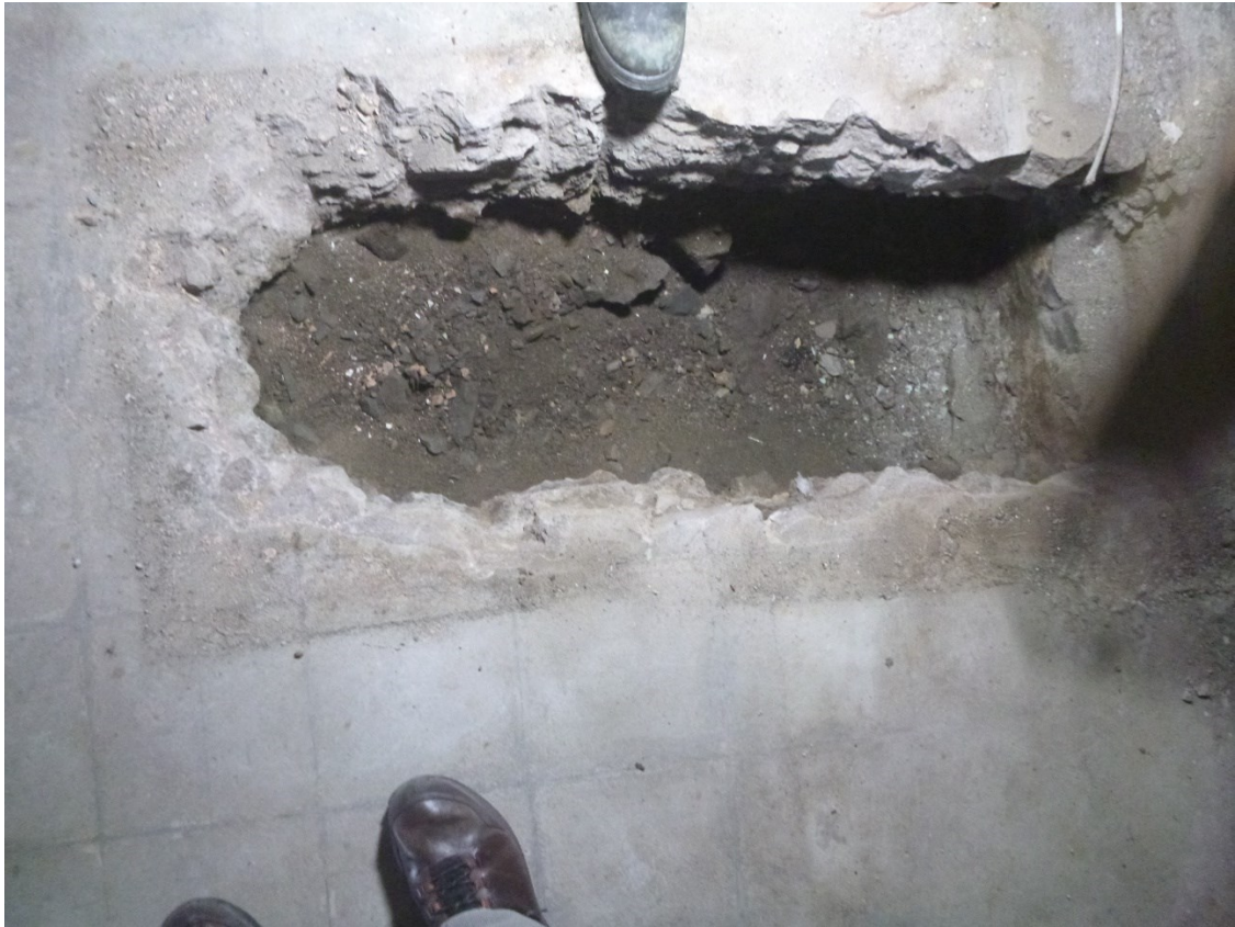
Photo 9: Trial hole in ground floor slab
