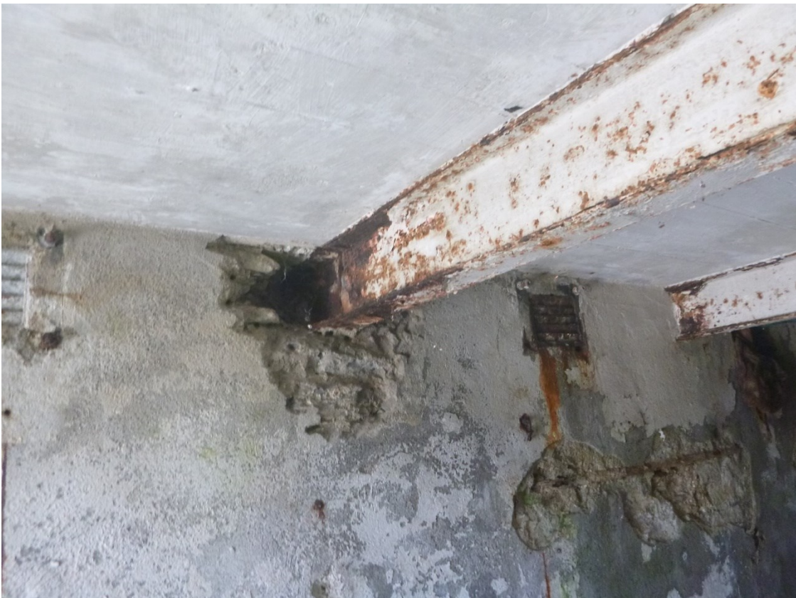
Photo 14: View of RSJ's supporting concrete roof slab of northern annex
