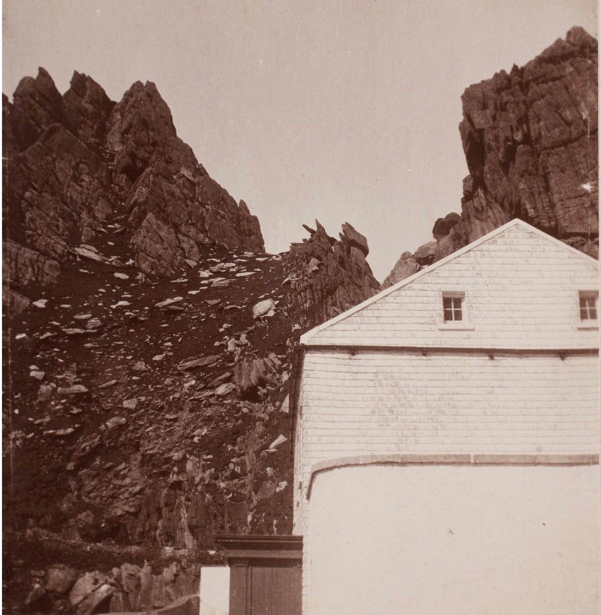
Photo 2: Archive photograph of original two storey building with pitched roof and slate cladding on external walls
