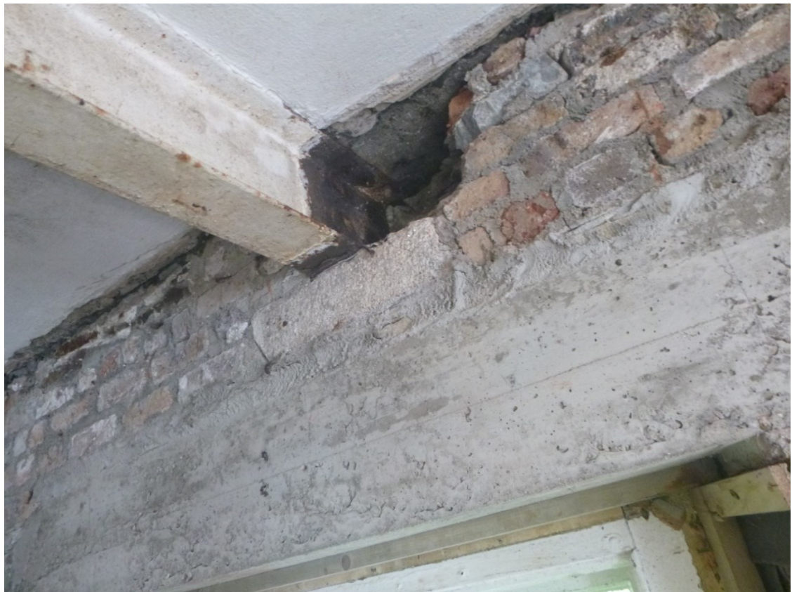
Photo 22: Roof RSJ bearing onto granite pad in rear wall
