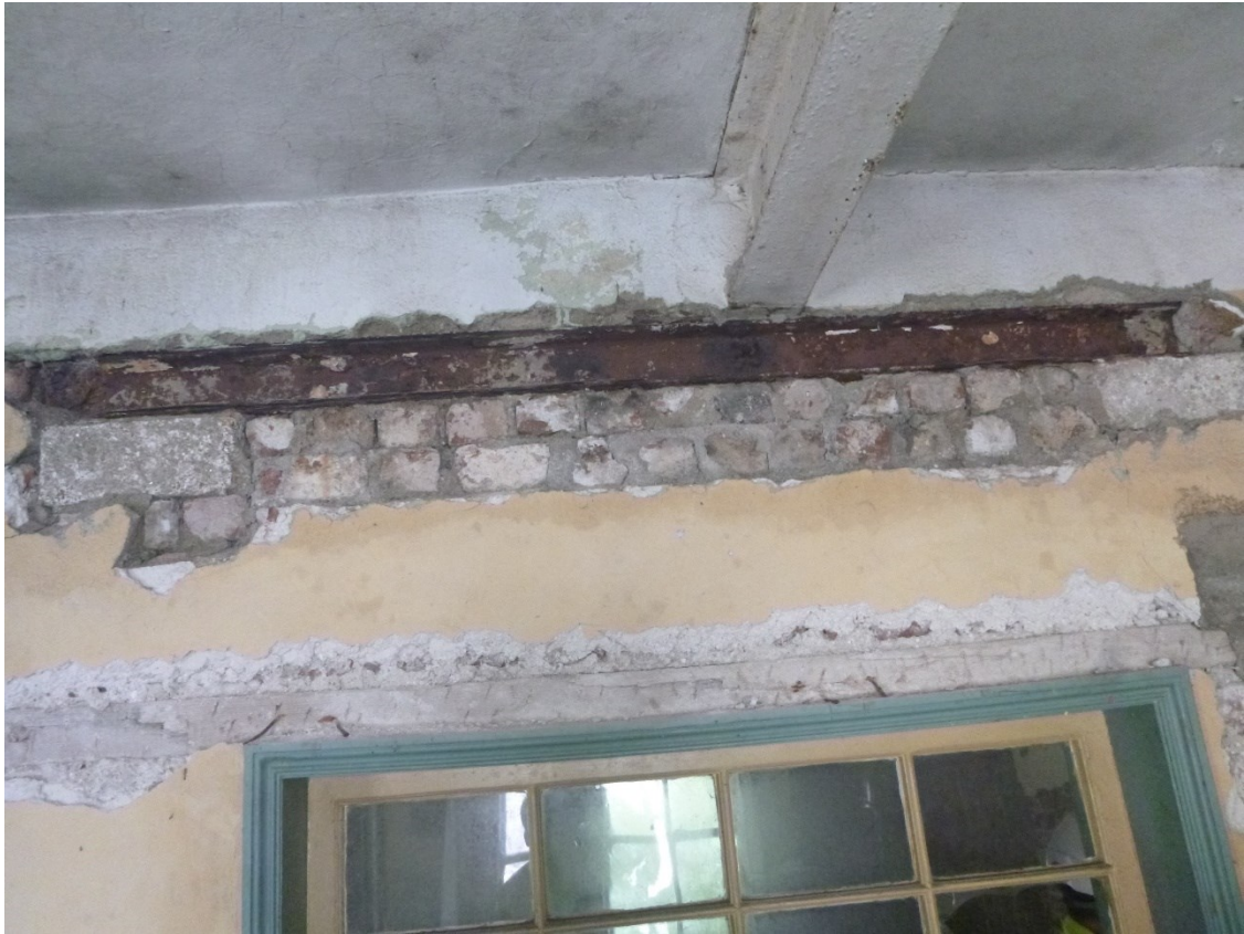
Photo 17: RSJ supporting roof slab bearing onto steel spreader in rear wall
