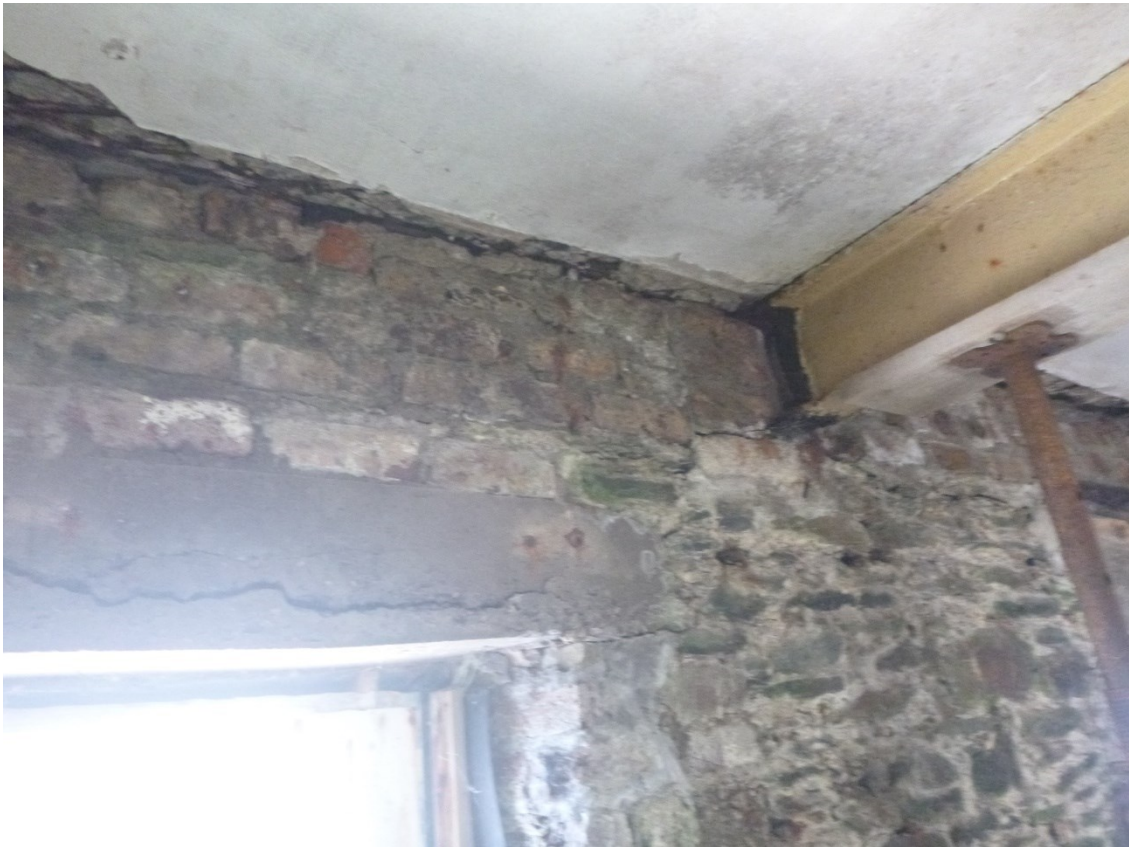
Photo 20: Propped roof RSJ bearing onto front wall
