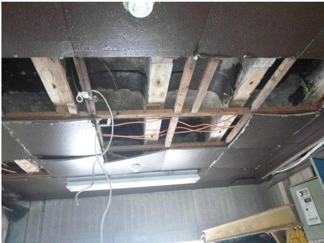
Photo 24: Underside of concrete rib slab roof of single storey machine room
