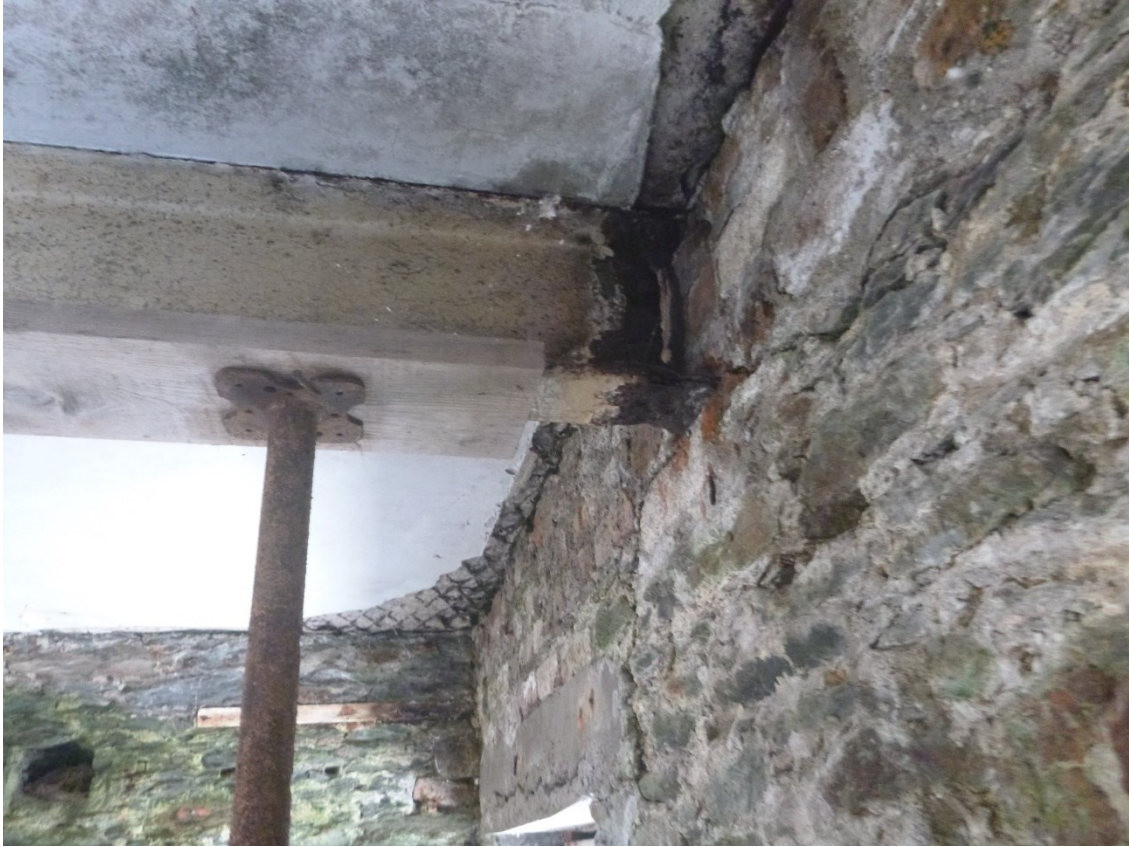
Photo 19: Propped roof RSJ bearing onto front wall
