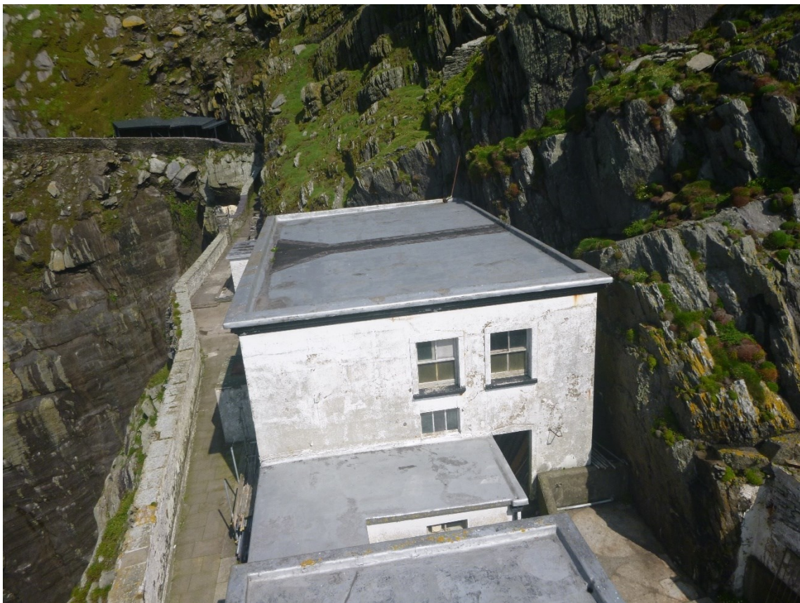
Photo 26: Flat roof of main two storey block
