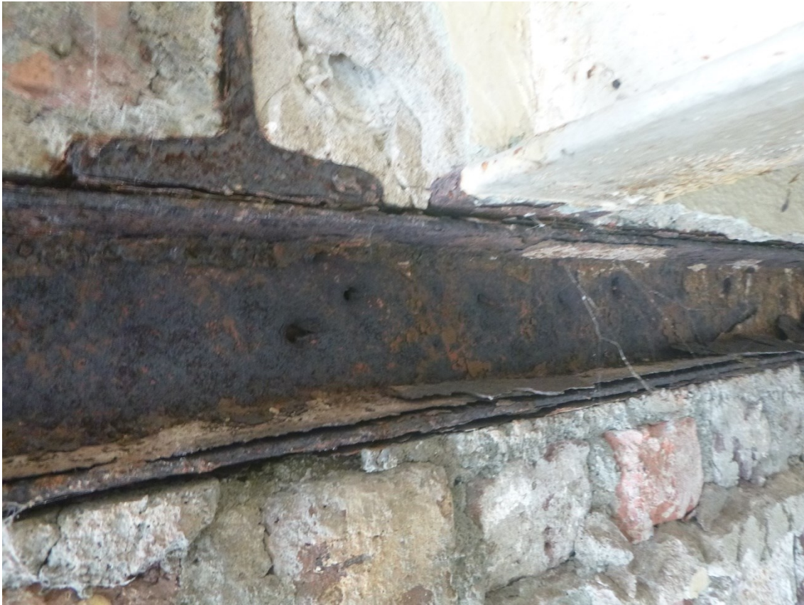
Photo 23: Roof RSJ's bearing onto steel spreader in spine wall
