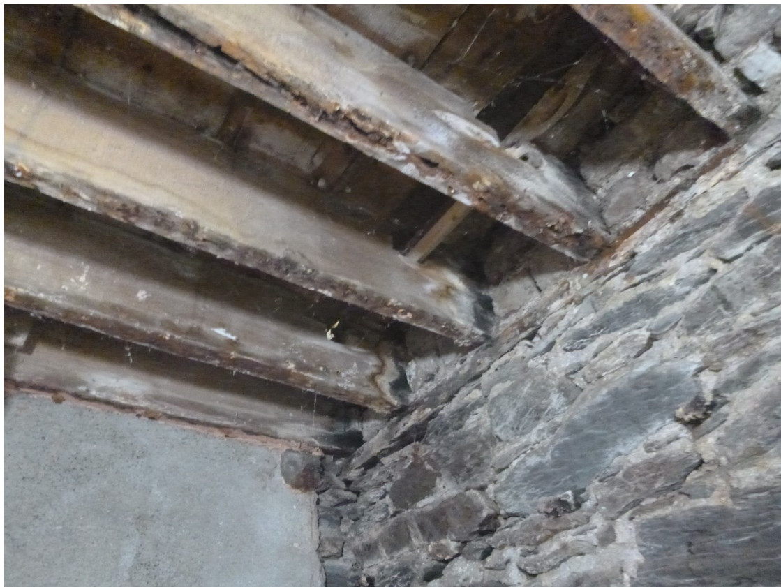
Photo 10: First floor timber joists built into front wall
