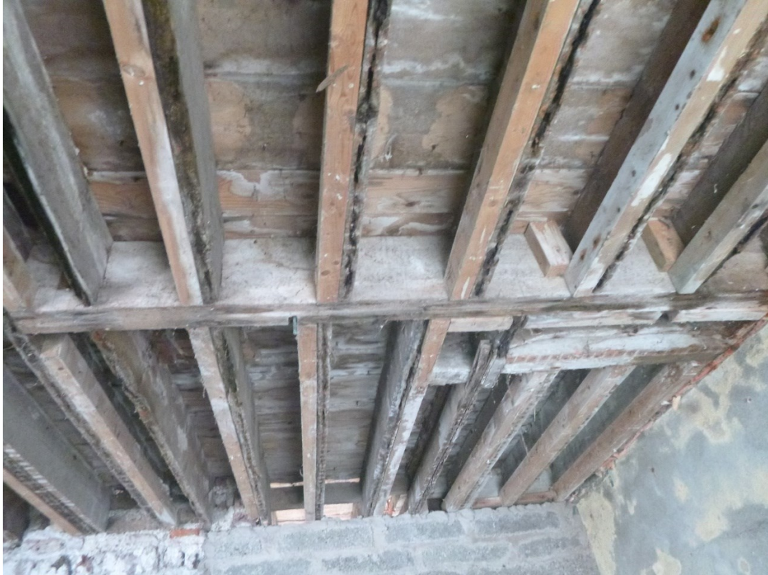
Photo 13: First floor timber joists trimmed around old stairwell opening
