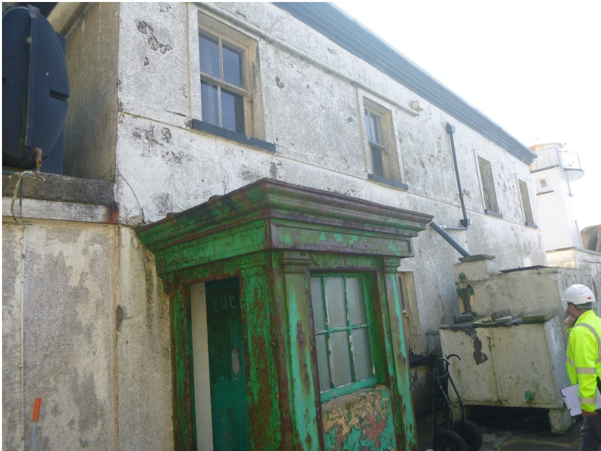
Photo 4: View of front (western) facade
