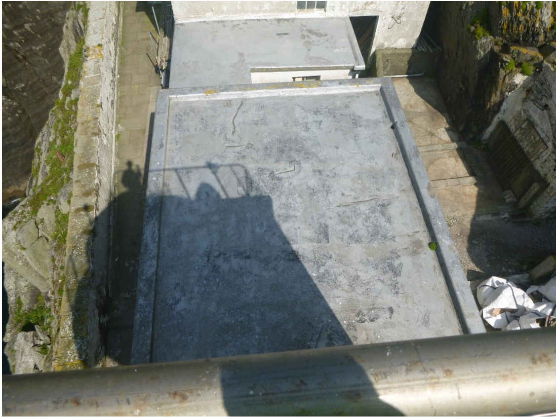
Photo 25: Roof of single storey machine room and entrance annex
