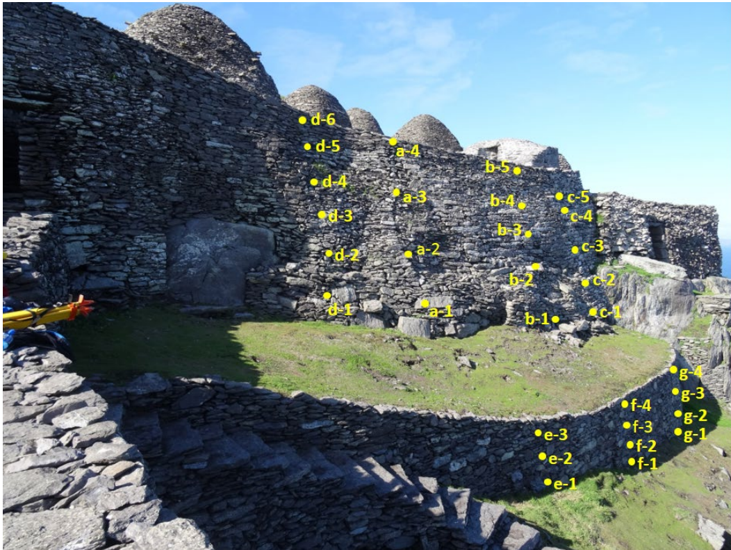
FIGURE 10 -SURVEY MARKERS IN AREA 2
