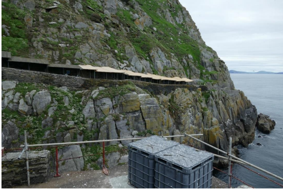
Figure 9 - View of the protective canopy on the Lower Lighthouse Road
