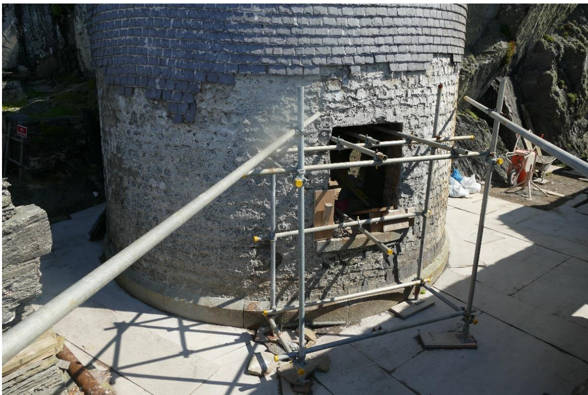
Figure 32 - View of the Upper Lighthouse Protection to floor slab.
