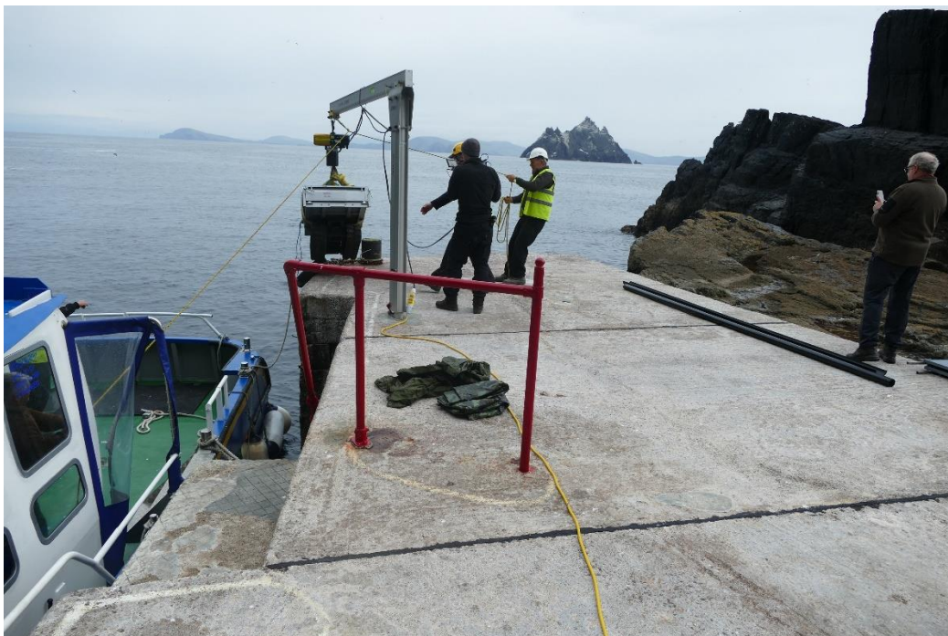
Figure 34 - View of the demountable hoist at the landing pier
