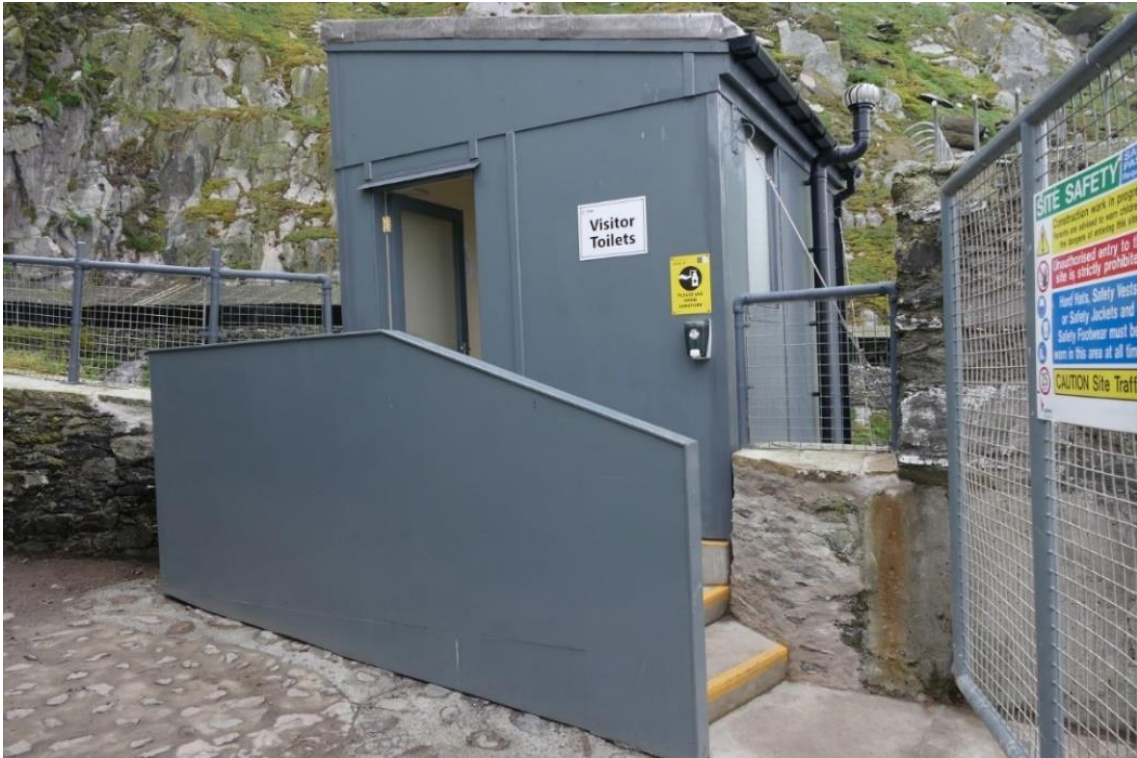
Figure 27 - View of the visitor toilets near the helipad
