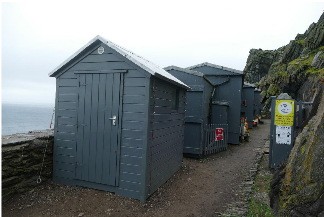
Figure 25 - View of the site huts on the Lower Lighthouse Road
