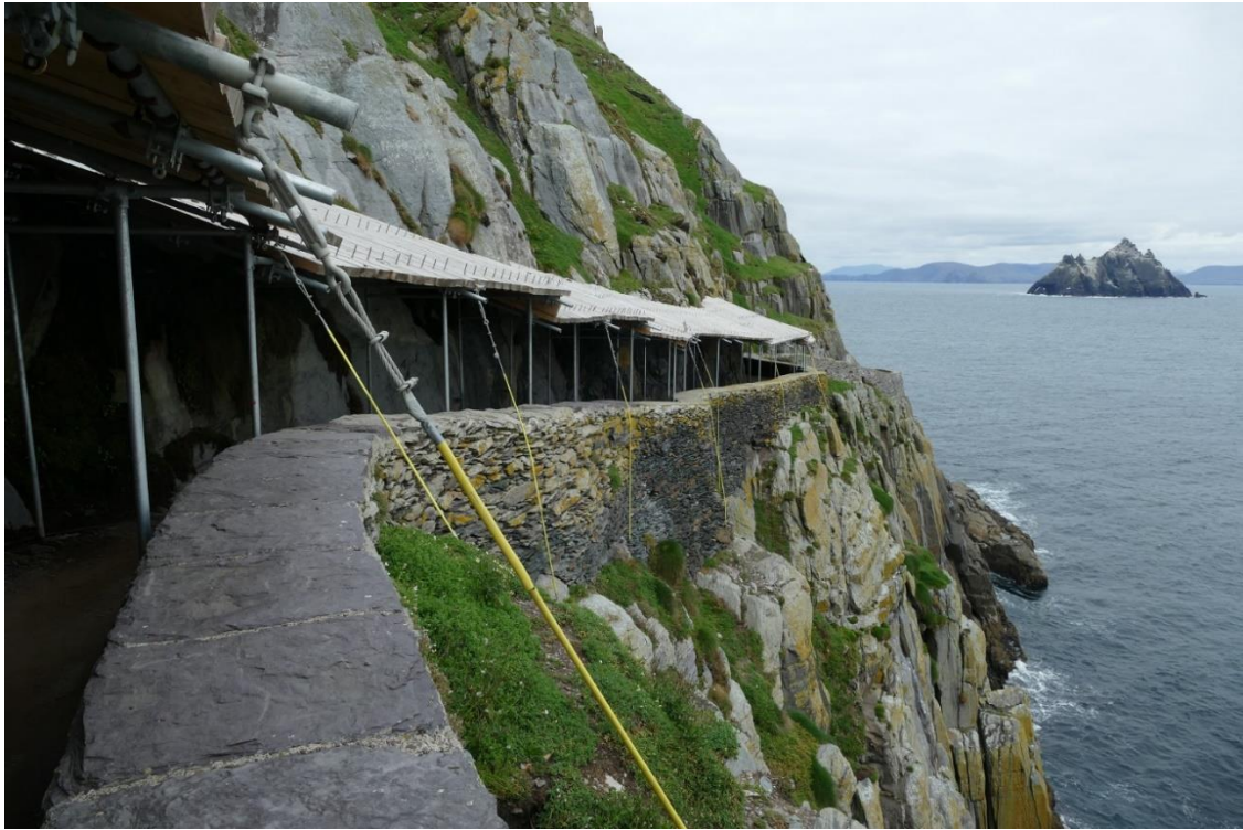
Figure 10 - View of the protective canopy on the Lower Lighthouse Road
