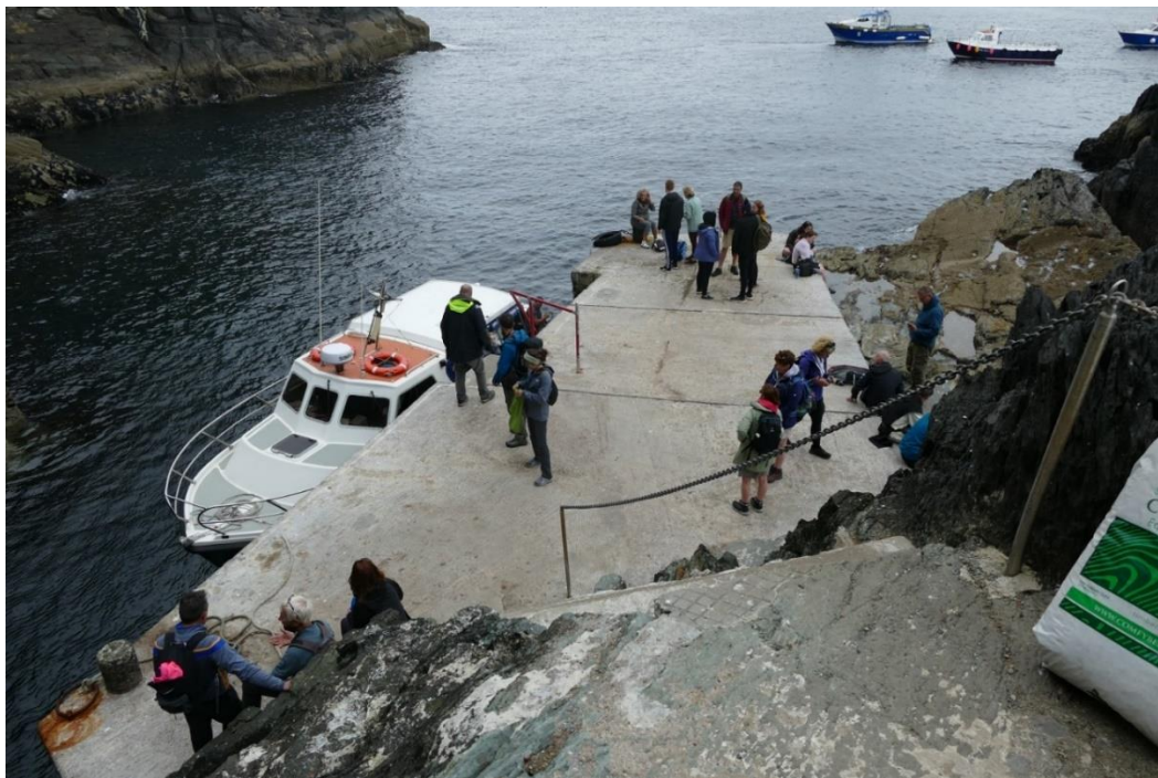
Figure 4 - View of the Landing Pier
