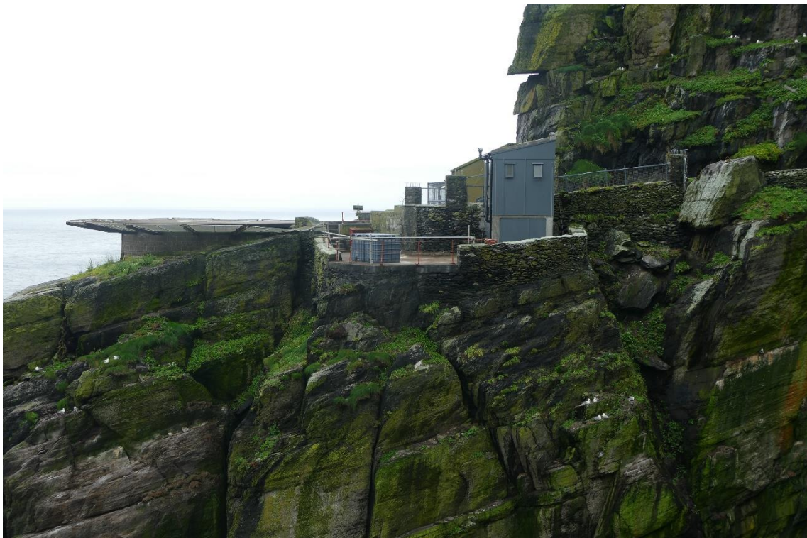
Figure 280 - View of the visitor toilets near the helipad
