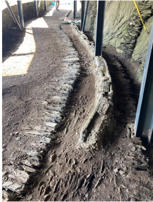
Fig. 14. Crash Deck 3, the reinstated features in its upper half.
