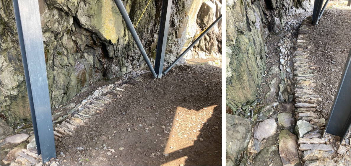
Figs. 5 & 6. Crash Deck 1, general views of the reinstated features.
