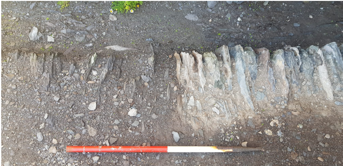
Fig. 10. Crash Deck 2, junction of original and reinstated road edging.
