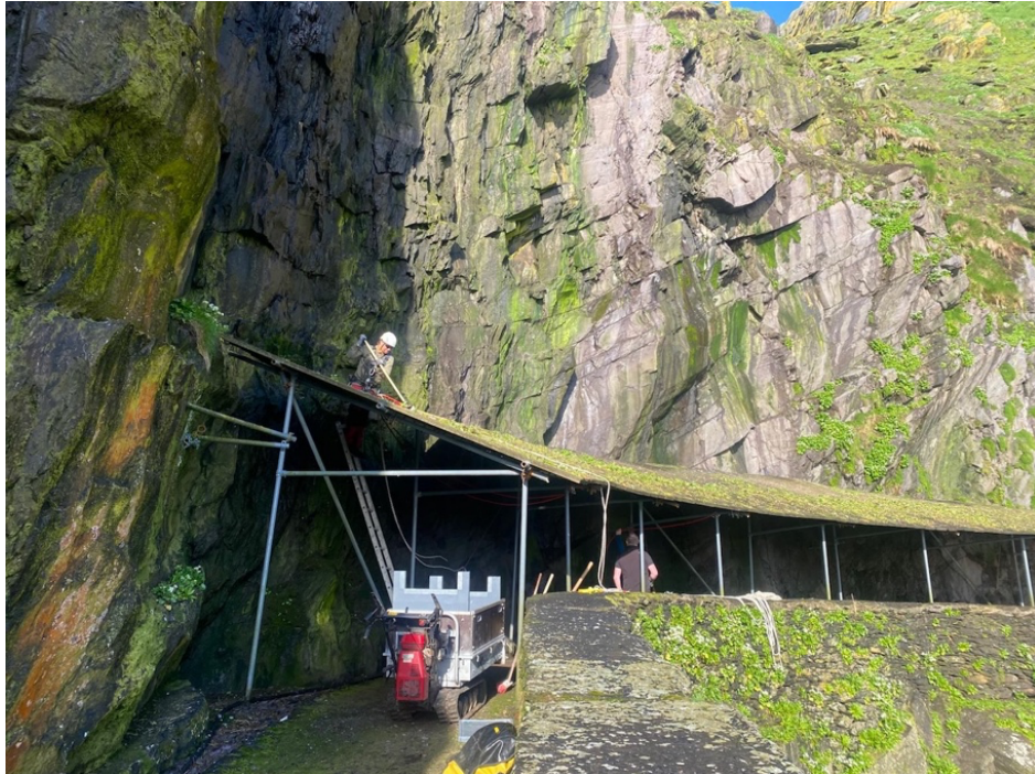
Fig. 4. Cleaning the original lighthouse-era canopy at Cross Cove.
