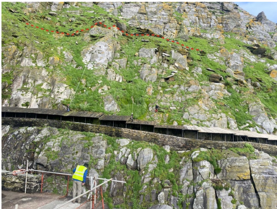
Fig. 3. Sweep lines 9-11 crossing the line of the East Link route (dotted red line)with ecologist monitoring work through telescope in foreground. The contrasting roofs distinguish the newer sections from the original lighthouse-era canopy over the lighthouse roadway.
