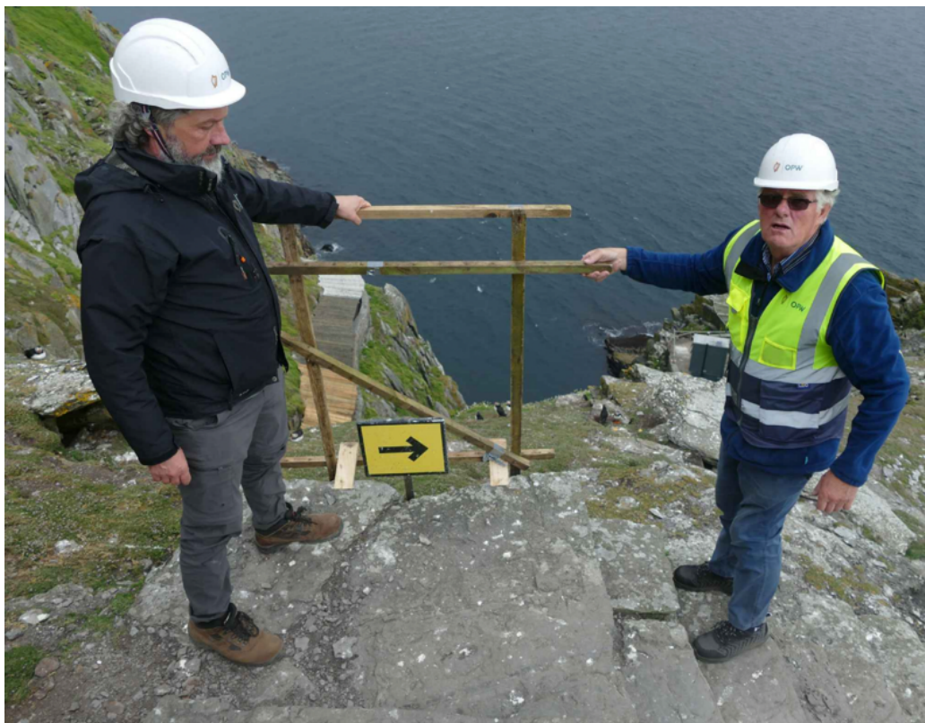
Fig . 3. Mock of the proposed barrier from the west illustrating the natural tendency for persons descending to lean on the proposed barrier (note tempting view down over Cross Cove) and also of persons ascending to hold onto it.
