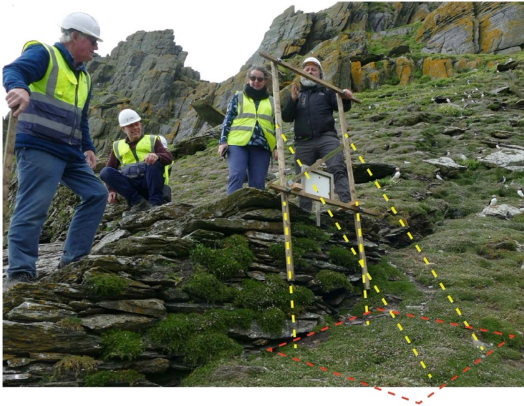
Fig. 4. Mock-up of the proposed barrier from the east with added yellow lines indicating base of uprights and possibly required raking braces and red lines showing likely area required to be excavated to accommodate anchoring of uprights and braces into bedrock.
