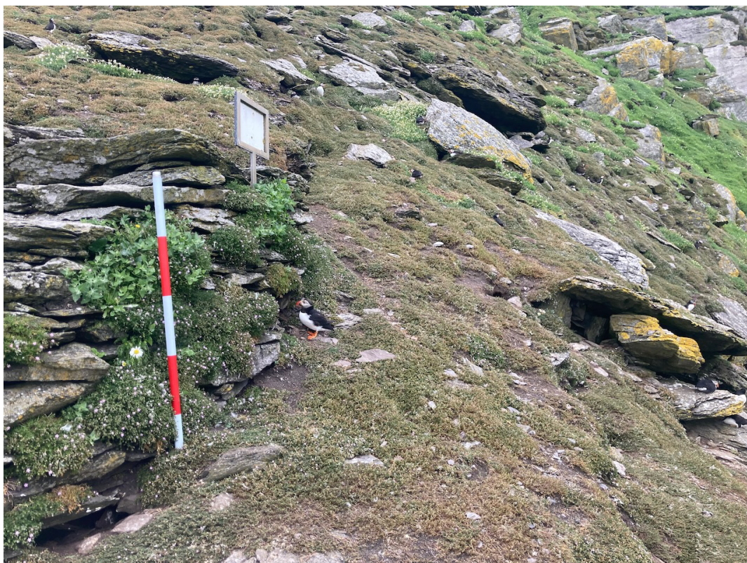
Fig. 2. The unnaturally looking flat area to the east of the corner of the South Steps (left) where it is proposed to erect the barrier. Could this be an early terrace? The puffin in the picture was guarding his / her nest in the base of the walling supporting this corner of the South Steps.
