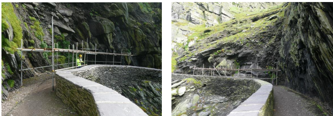
Fig. 36. – Temporary crash deck location B & C on the Upper Lighthouse Road.
