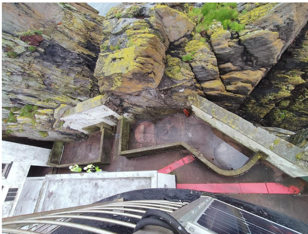
Fig. 13. – Area in the Lower Lighthouse Compound where former fuel tanks were removed
