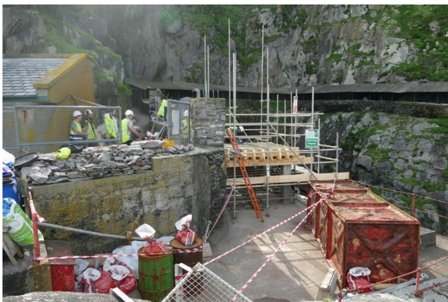
Fig. 23. – Construction of the concrete base prior to the installation of the visitor toilets
