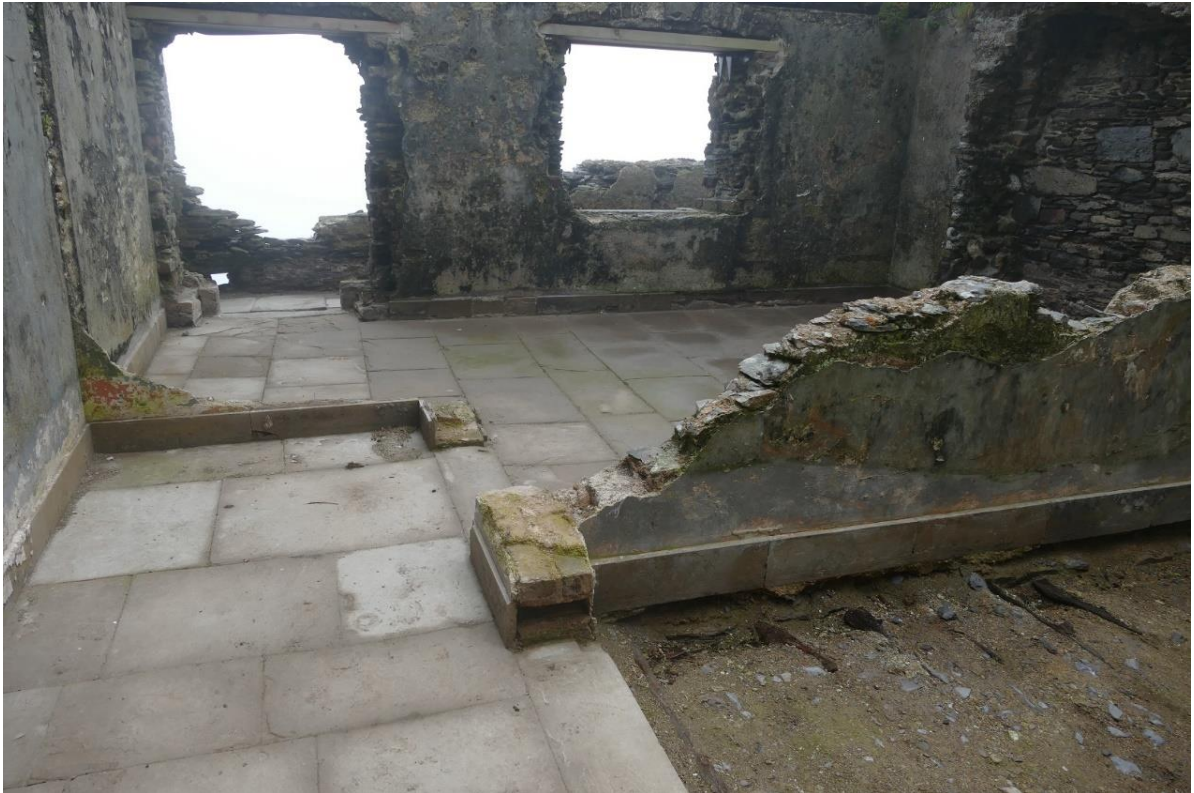
Fig. 19. – Exposed sandstone flooring at the Upper Lighthouse
