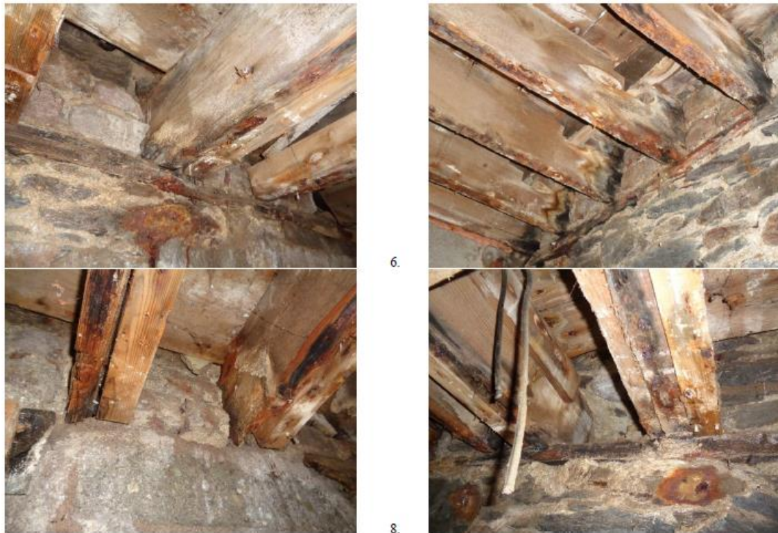
Fig. 15. – Existing timbers in poor condition at the Lower Lighthouse. Ref. Appendix F.
