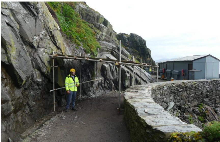
Fig. 35. – Temporary crash deck location A near site huts and installed following rock-fall.
